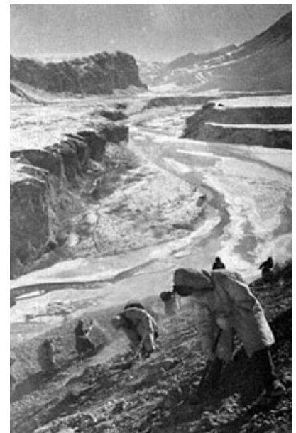
Construction of the canal between the Dniepr and Boug rivers. 1935.
