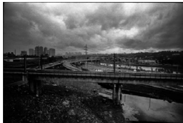
Rivers were silted by garbage and debris after the typhoon.
